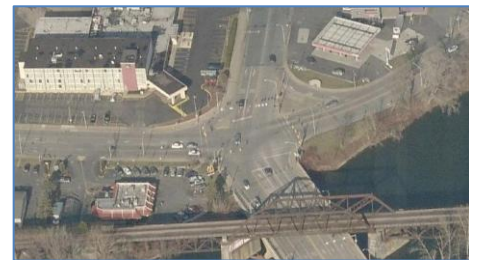
The intersection of 3 rd St. & Larry Holmes Drive
